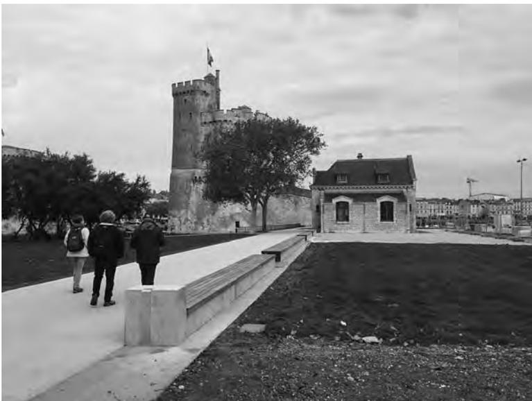
[fig. 4] Integration of anti-submersion systems into the public spaces of the La Rochelle old harbour.
