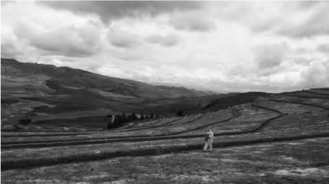
[fig.2] Geotechnical stabilization in progressive closure of La Quinoa Pit in Yanacocha mine, Cajamarca 2015. Re-filling, top-soil installation and row plantation of rice bales for erosion prevention. Source: photographed by the author.
