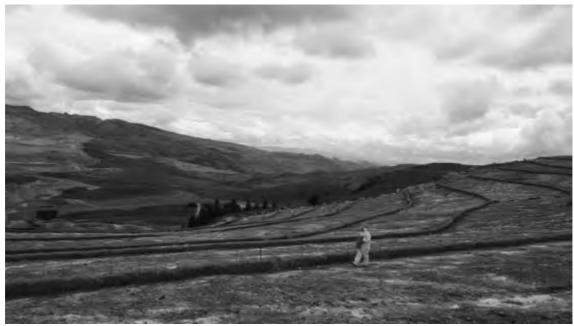
[fig.2] Geotechnical stabilization in progressive closure of La Quinua Pit in Yanacocha mine, Cajamarca 2015. Re-filling, top-soil installation and row plantation of rice bales for erosion prevention. Source: photographed by the author.
