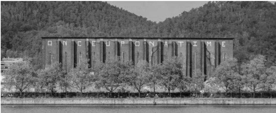
Above: The former patinoire de Liège, also known as the Palais des fêtes de Coronmeuse (J. Moutschen) was built for the 1939 International Water Exhibition and later used as an ice rink. It stands vacant since 2012 and is threatened with demolition.
