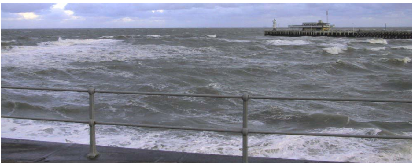
Fig. 1. Waves propagating in the shallow water area between Zeeheldenplein (front) and Western pier (background), near the measurement site in Oostende.
