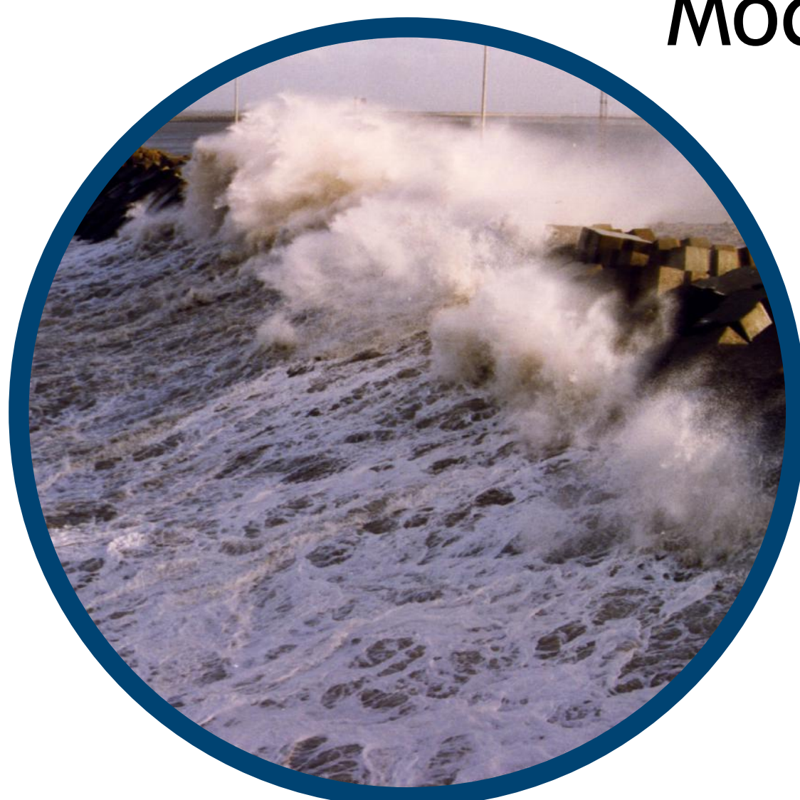
Coastal & Offshore Structures
