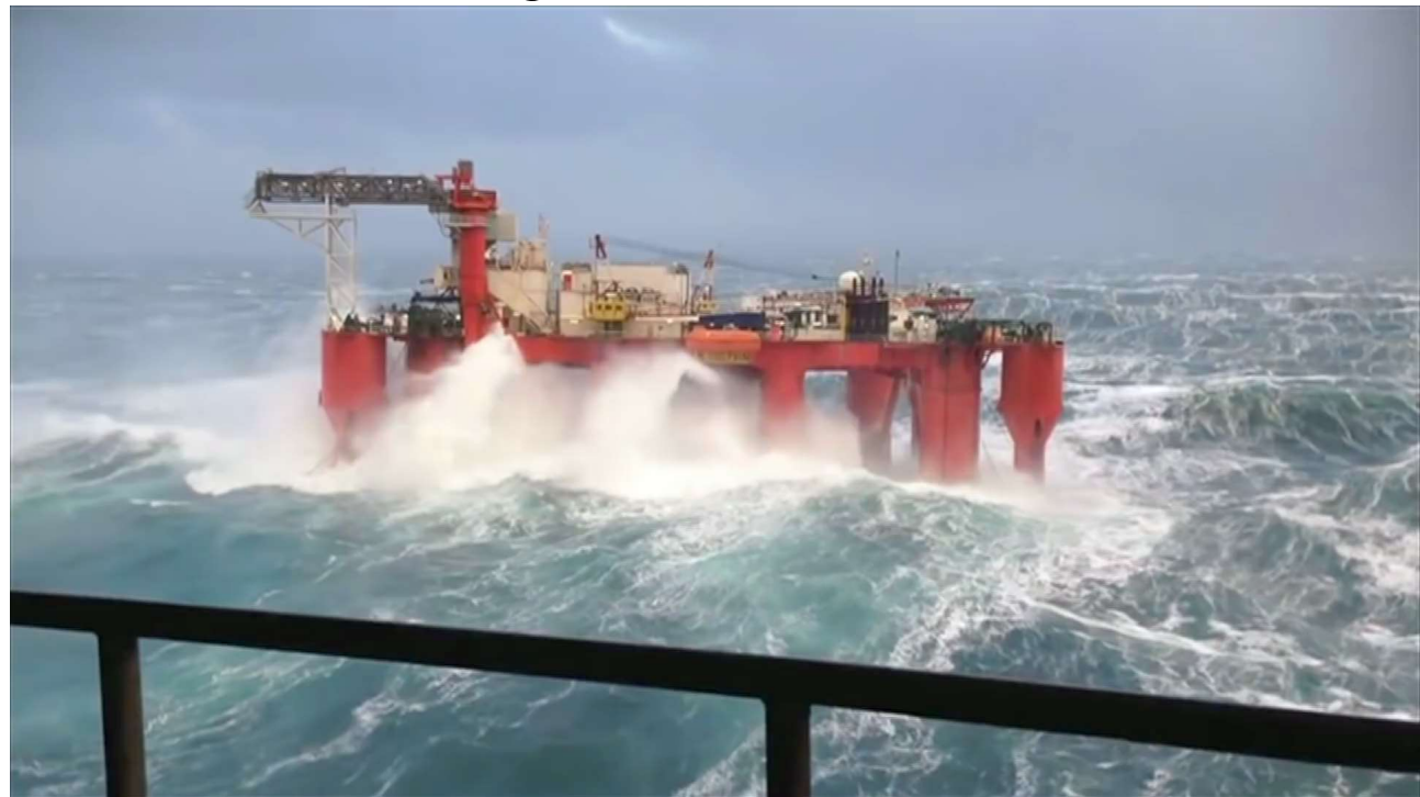
Huge wave impact on a ship, offshore platform,...
