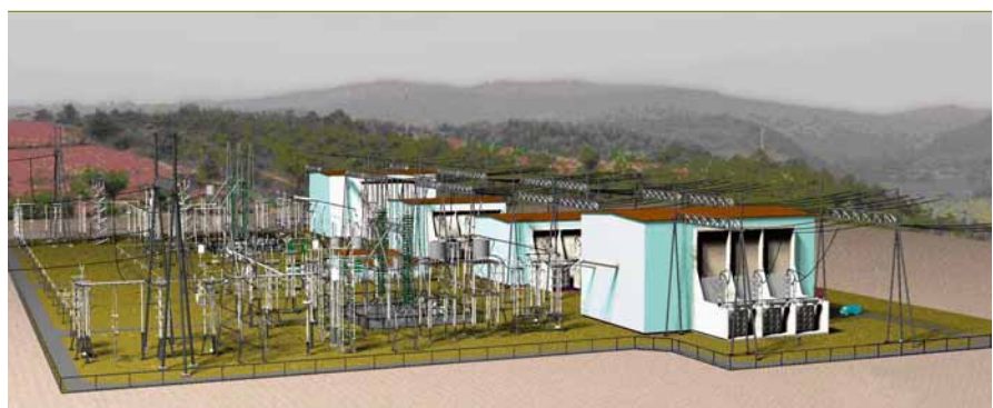
A computer-generated illustration of an 800 kV converter station
