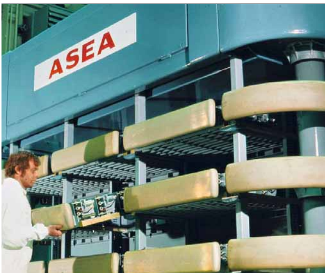
An early ASEA thyristor-based HVDC converter
