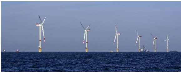
Figure 1: Wind turbines D1 to D6 of Thorntonbank Wind Farm (C-Power).
