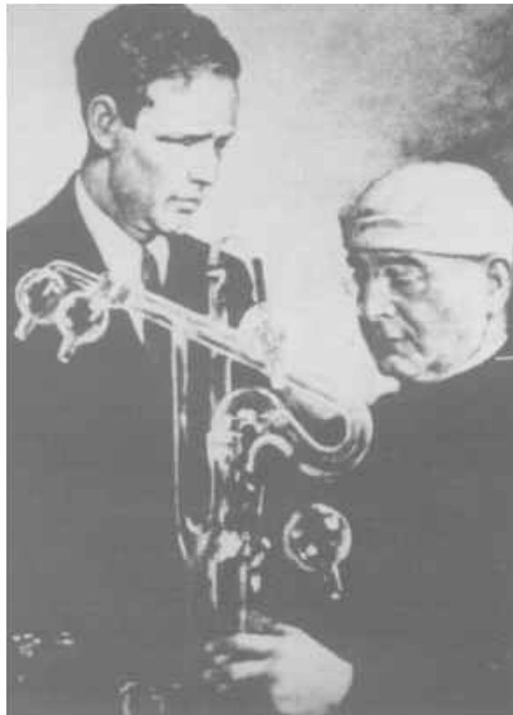
Figure I.6: Charles Lindbergh and Alexis Carrel with the first pump oxygenator. <71>
